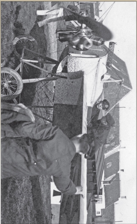
Gottard Sachsenberg test runs the Oberursel U.I engine of Fokker E.III 1F196 at MFA 2 (Marine Feld Abt. 2) in 1916. Sachsenberg would go on to score 31 victories before the Armistice, although none of these were while flying a Fokker Eindecker. Note the uncovered wire wheels.
